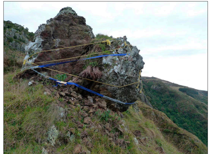
Trussed boulder above Faulkner's Track. Ohinetahi Reserve remains closed—safety of our volunteers and public users is paramount!
