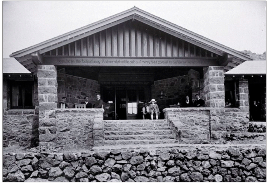
Afternoon tea at the Sign of the Kiwi tearooms, circa 1925. An example of a dry stone wall features in the foreground, many of these well-made walls still exist today. During the depression, a similar wall adjacent to the Sign of the Takahe became the subject of heated debate later in the story.
