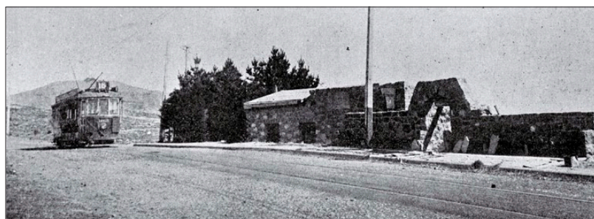
The Sign of the Takahe during construction phase, circa 1922–25
