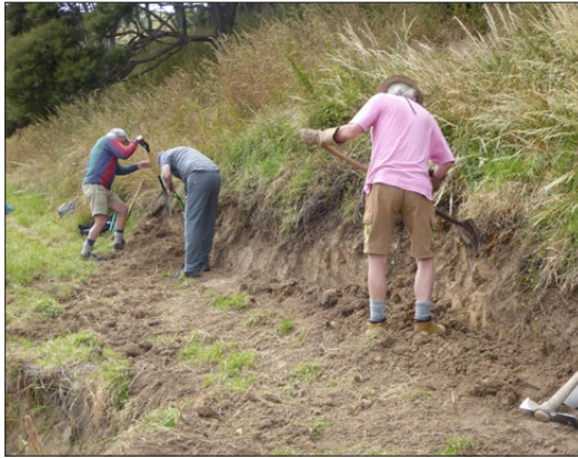
The team hard at work widening Rhodes Track
