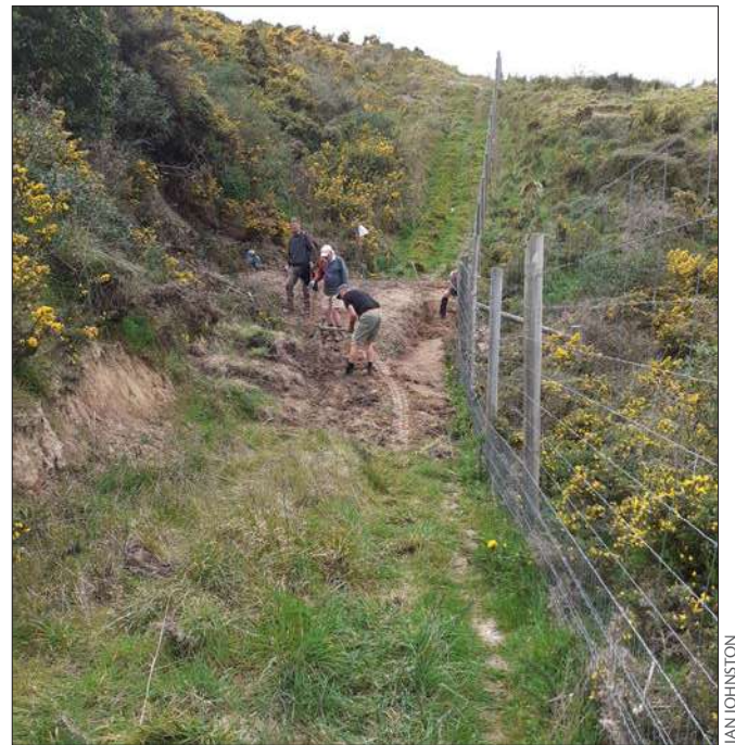
Volunteers repairing one of the minor slips on the boundary
