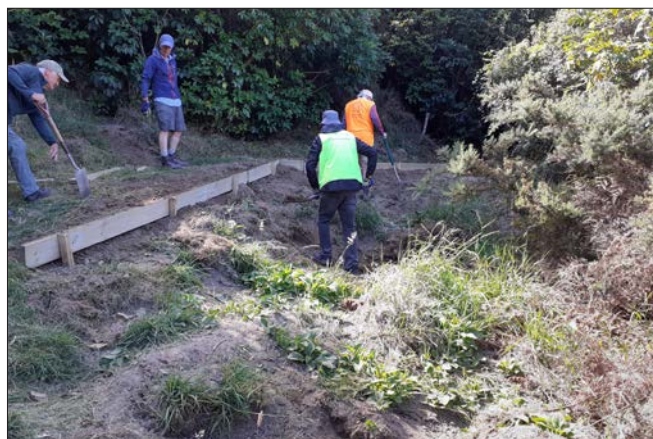
Omahu work party undertaking repairs to Kirks Track
